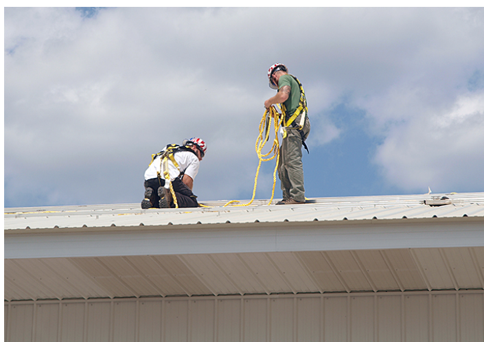
Installers from the Radiant Store in Troy, NY get a roof ready for solar thermal. (Photo courtesy: NYSERDA)
